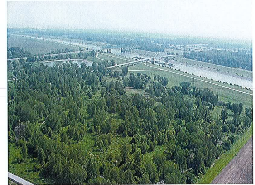
Canal and I-270 Bridges
