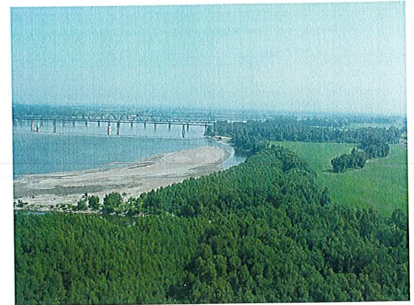
View of Bridge Complex Looking North
